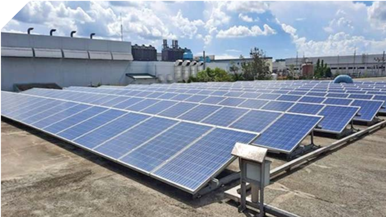
Laguna Water's onsite solar panels have a capacity of 57 kWp that provide clean energy and contribute to lower carbon emissions.
