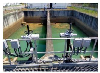
To further reduce water withdrawal, the East La Mesa and Balara Treatment Plants recovered and reused 3.813 mcm of backwash water to add to the production of potable water. East La Mesa Treatment Plant recovers and reuses 100% backwash water.
