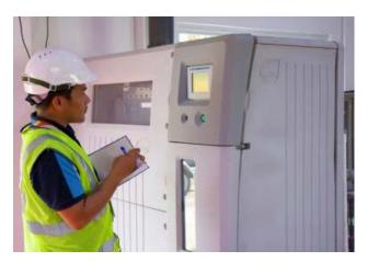
At the Laguna Water Wellfield, we employ MIOX technology that uses salt as a raw material for the onsite production of liquid sodium hypochlorite. The shift to this technology improved our chemical efficiency and the reliability of chlorine supply.
