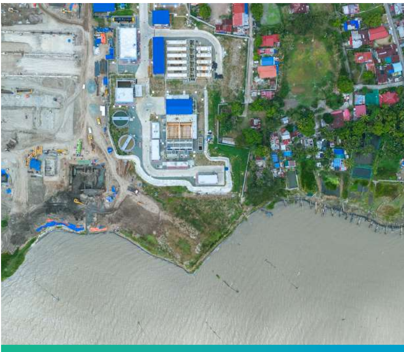
The East Bay Water Treatment Plant is our second facility that abstracts raw water from Laguna Lake, providing additional water to the East Zone.
