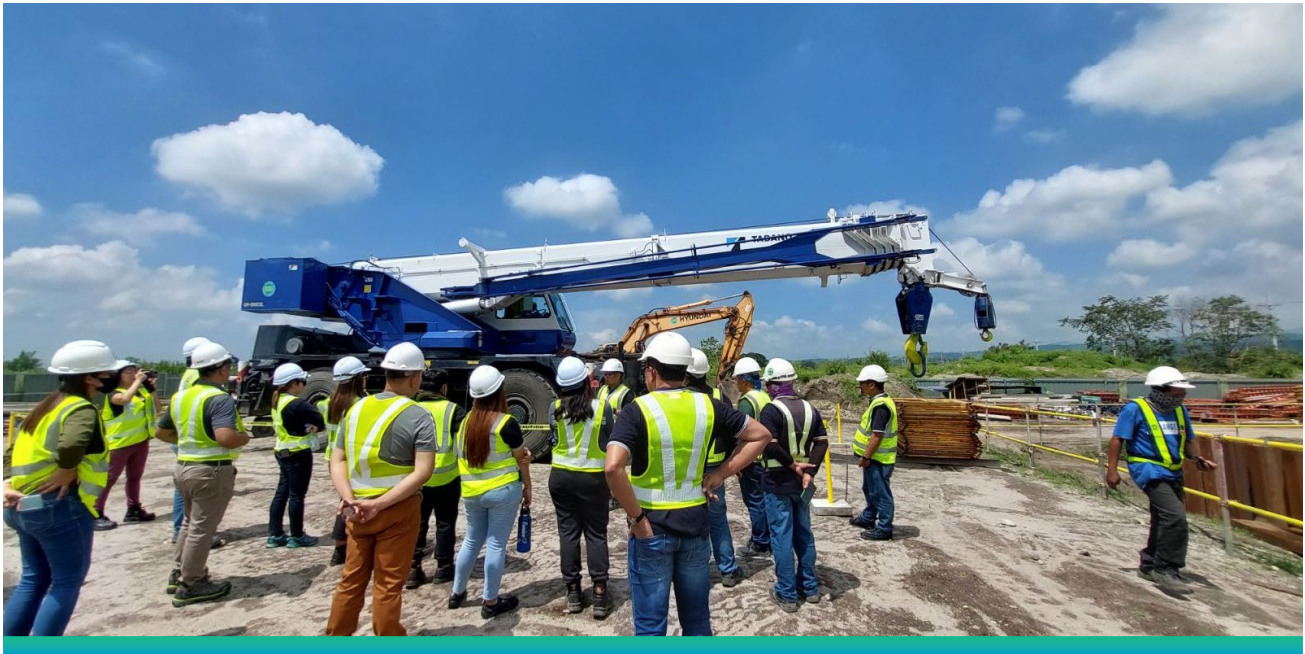
This safety walk-through at our site in Pampanga is just one of the many conducted regularly, aiming to identify potential safety hazards, assess the status of safety in the workplace, and provide feedback to personnel on proper safety practices.
