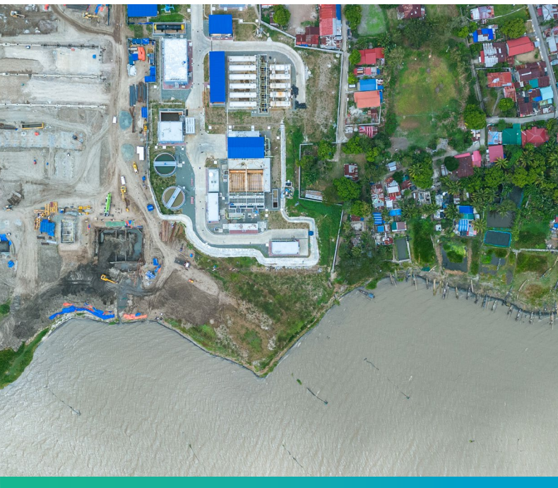
The East Bay Water Treatment Plant is our second facility that abstracts raw water from Laguna Lake, providing additional water to the East Zone.
